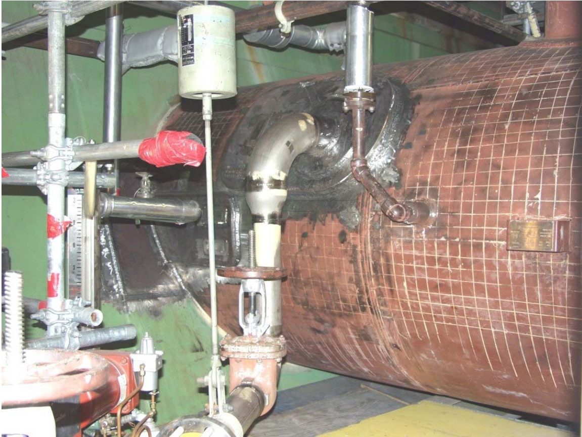
Completed PMCap Installation
